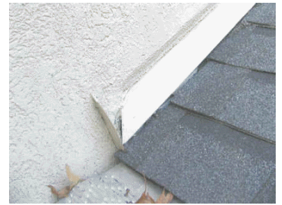
Kickout flashing failing.
